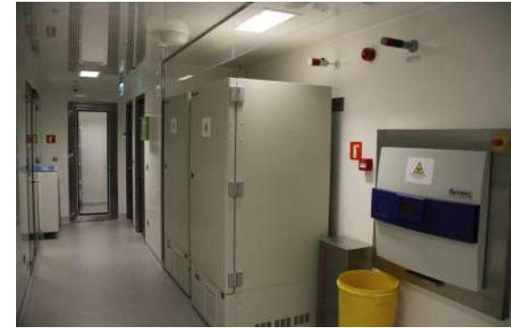
BSL-3 Main Hall, Storage and Cold room
